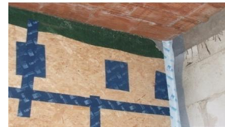
Taping off the OSB boards, and connection between OSB and plaster on the brick walls (the white band in the upper photo)
